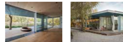
Detached house Freiburg, DE Ref. 1447*
